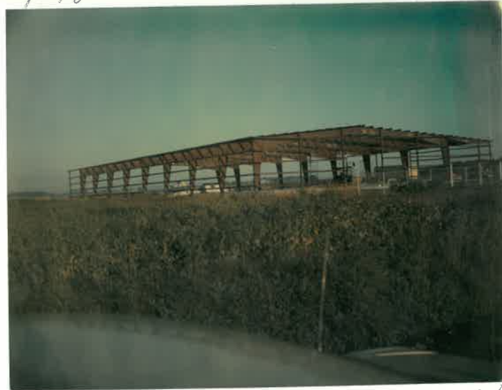
SERVICE BUILDING R/L
